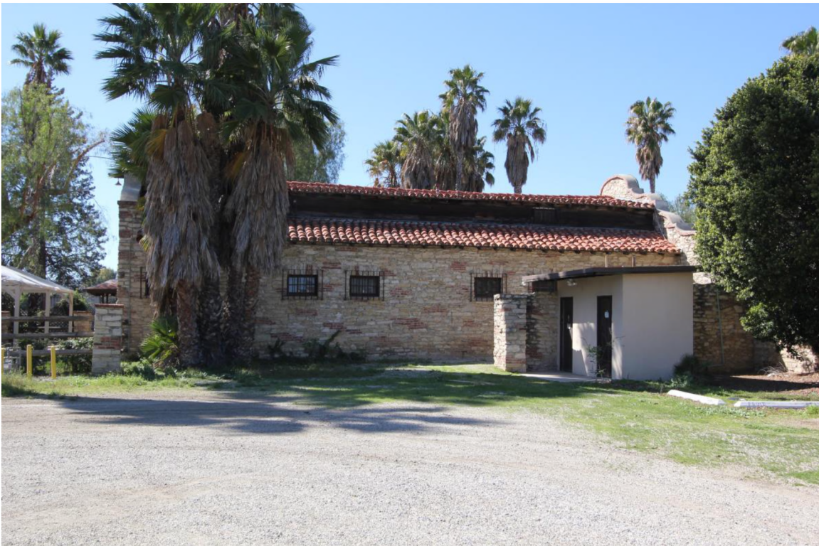
Figure 13: View showing the break in the roof line that roughly corresponds to the second floor attic space, view west, 2016 (Chattel, Inc.)
