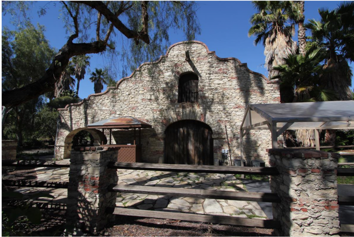
Figure 10: Canoga Mission Gallery, view north, 2016 (Chattel, Inc.)
