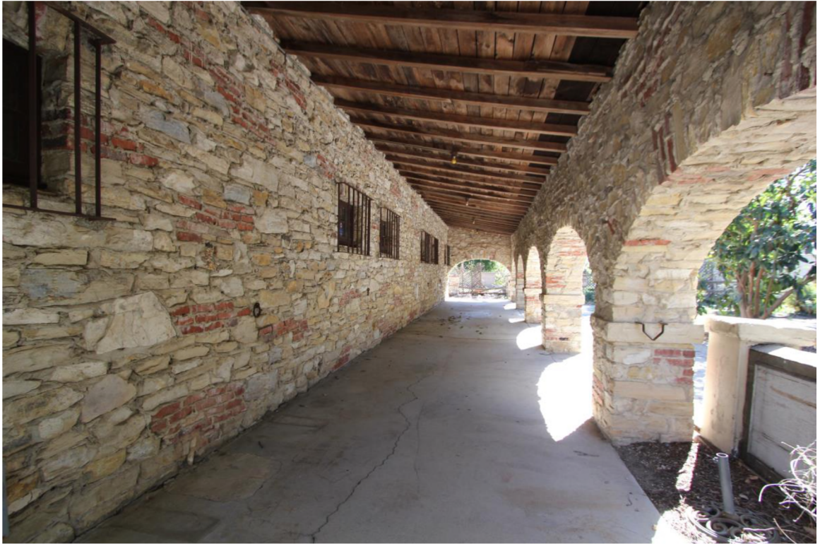
Figure 9. Canoga Mission Gallery, West bay loggia, view south, showcasing the use of stone and brick with weeping mortar used throughout the Canoga Mission Gallery, 2016 (Chattel, Inc.)
