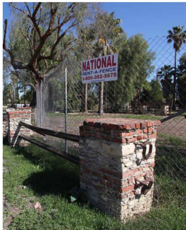
Figure 7: Detail of the historic stone and brick pilasters with wood split rail fence associated with the Canoga Mission Gallery, 2016 (Chattel, Inc.)
